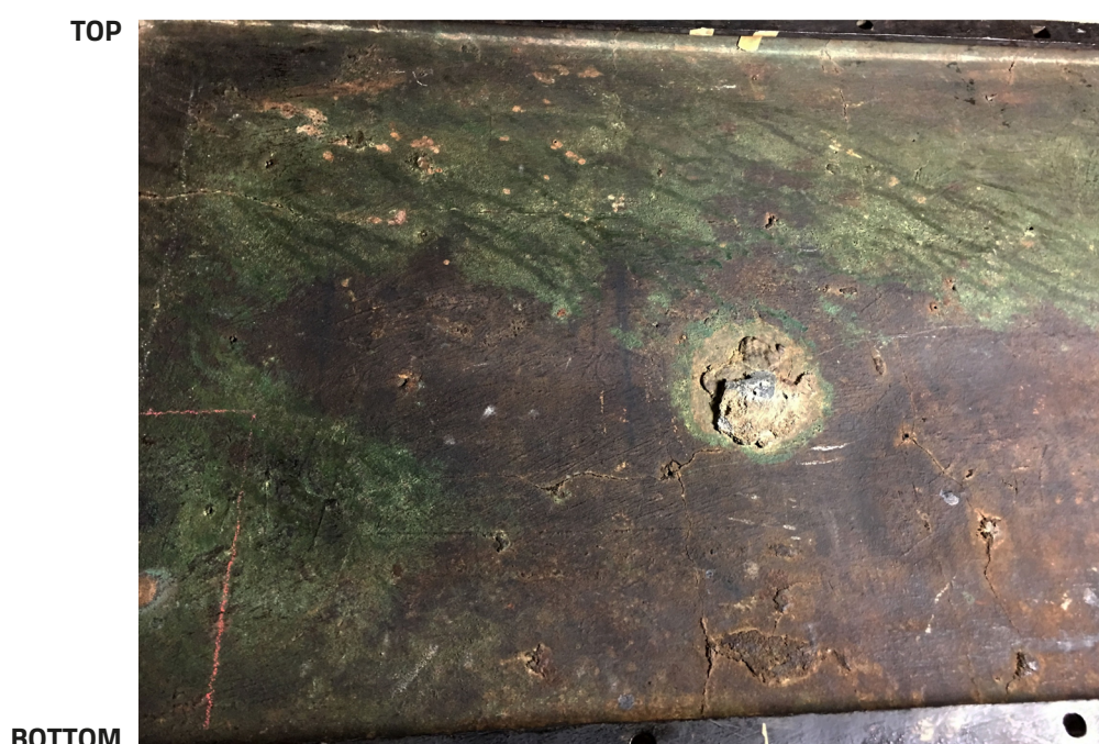
Fig. 26: Underside of the Mensa, showing drip marks, evidence of exposure to water. Photo by the authors.
